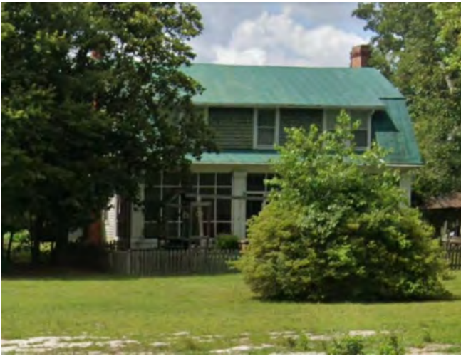
North-facing view of the Stuart Vann Bowen House (PD0081) located in the northern portion of the Site, off of NC-53.
