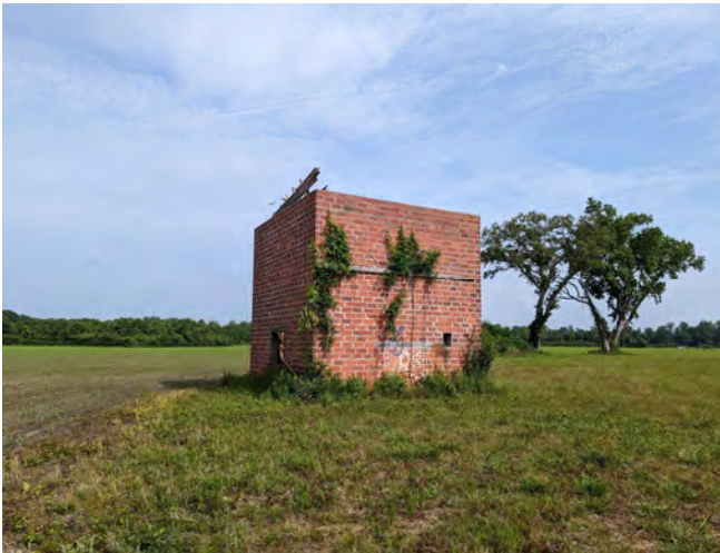
North-facing view of abandoned brick structure in the northern portion of the Site.
