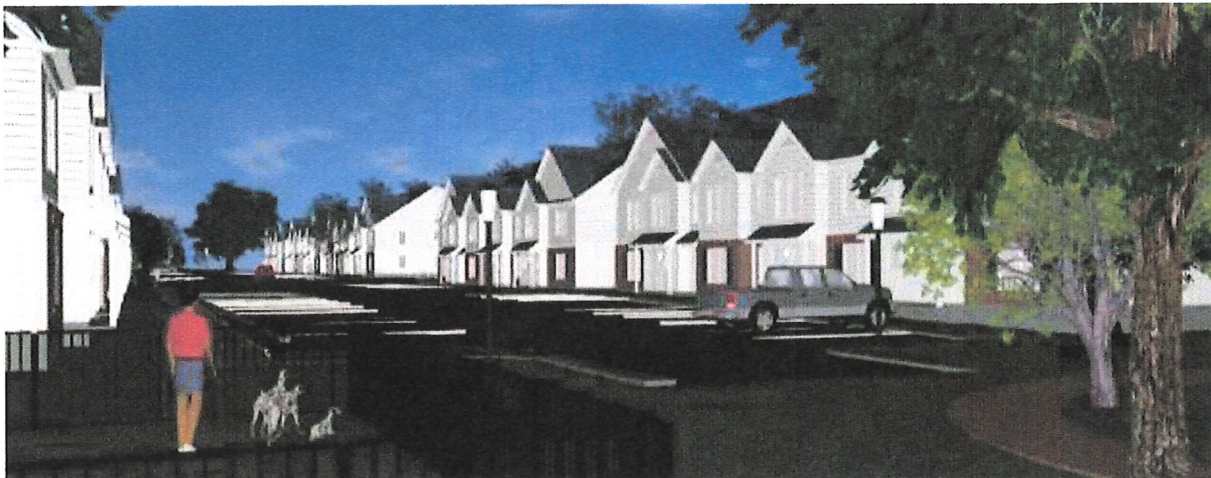
Exhibit 7.5 View From Rear of Project Source (Town of Burgaw Planning Board Case Summary)
